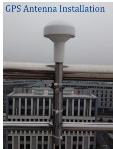
The server consists of the outdoor part and interior part. The outdoor part is composed of the GPS satellite receiving antenna, lightning arrester and antenna amplifier (optional). The function is to complete the reception of satellite signals.
