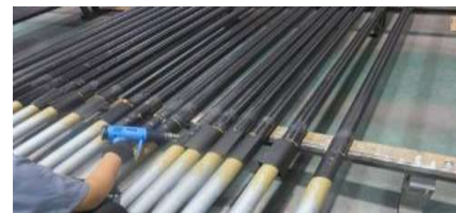
锚栓防腐和密封
